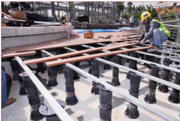
VersiJack® provide stable support for installation of decking
