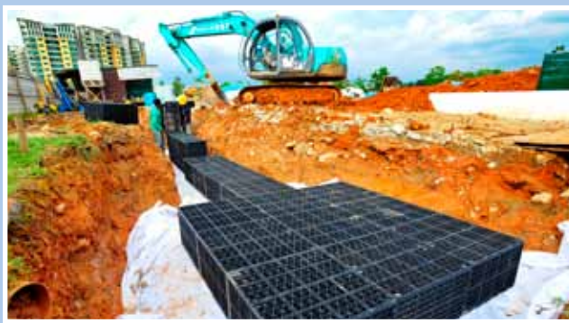
VersiTank® Infiltration System installed at a park
